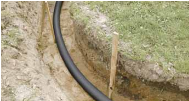
Fig. 47 Laying a bend area
