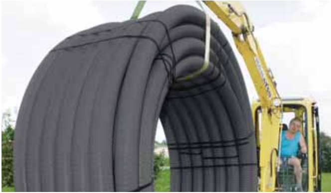
Fig. 40 Lifting with a digger
