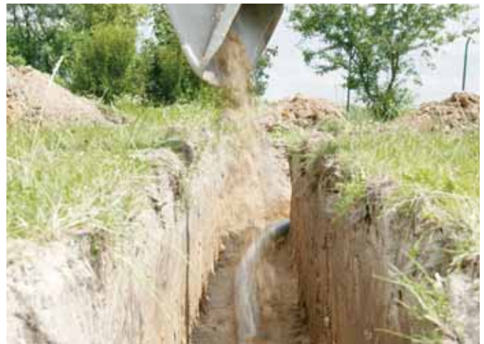
Fig. 49 Backfilling trenches with sand
