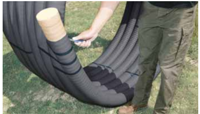
Fig. 44 Cutting the coil straps
