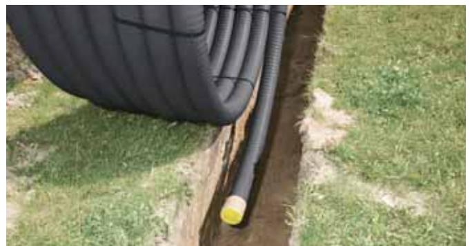
Fig. 45 Opening the coil layer by layer
