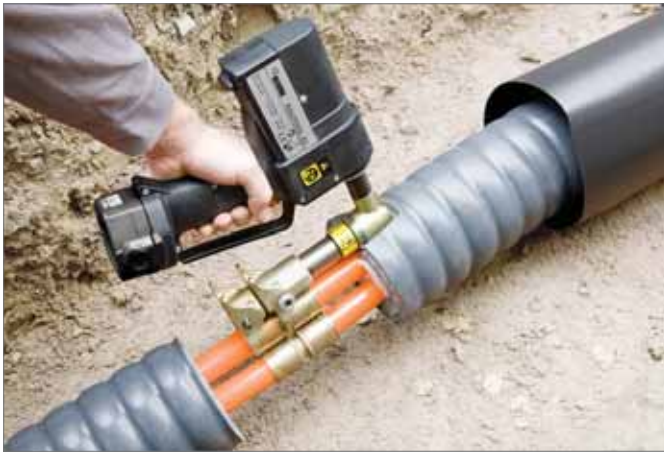
Fig. 2 RAUVITHERM compression sleeve joint
