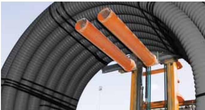
Fig. 41 Lifting with a forklift
