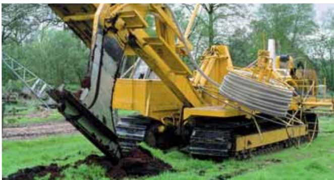
Fig. 29 Ploughing-in technique
