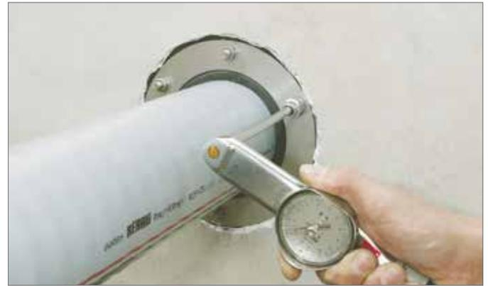
Fig. 5-14 Assembly with a torque wrench
