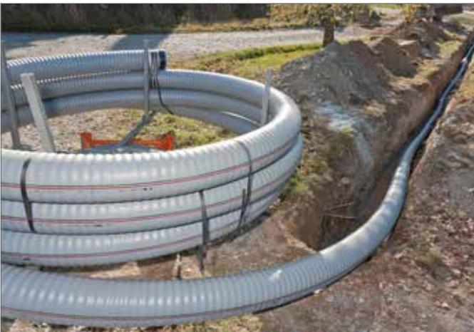
Fig. 7-29 Stationary horizontal unwinding device at the end of the trench
