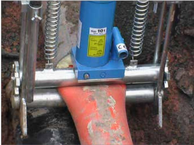
Fig. 7-26 Squeezing UNO carrier pipe
