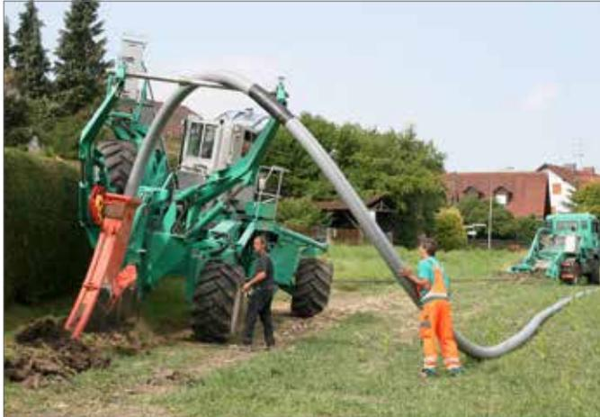
Fig. 7-8 Installation with a pipe plough
