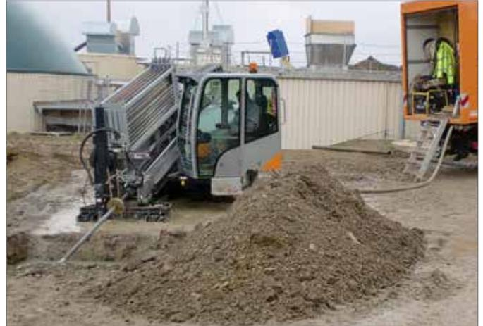
Fig. 7-10 Installation with horizontal directional drilling unit
