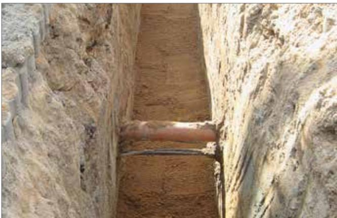
Fig. 7-2 Pipe trench with pipe support
