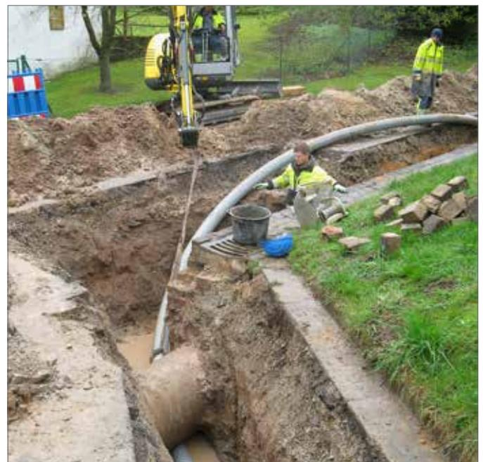
Fig. 7-21 Simple installation due to the flexible pipe routing
