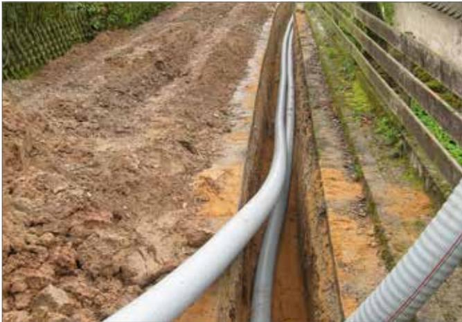
Fig. 7-4 Installation with the open-cut technique
