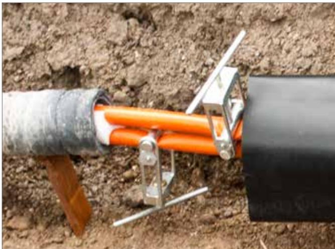
Fig. 7-27 Squeezing DUO carrier pipe
