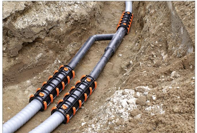
Fig. 4-23 Y-pipe installation in practise
