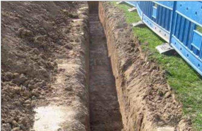
Fig. 7-1 Suitable trench base
