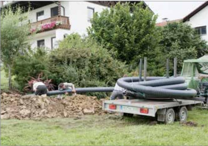
Fig. 7-28 Mobile horizontal unwinding device on a trailer
